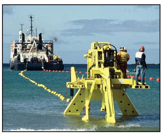
A plough being prepared to start the burial of a cable Source: Seaworks, NZ
