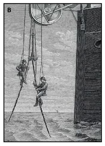
[A] Cable ship trailing grapnel to retrieve cable followed by [B] securing of the cable ready for repair Source: Traité de Télégraphie Sous-Marine by E. Wüschendorff, 1888
